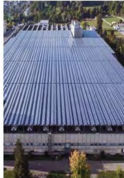
36'000 m 2 (5 football fields), 5 GWh/a Riverside in Zuchwil, 2015
