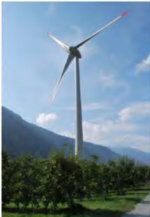
2 MW wind turbine, 5 GWh/a RhoneEole Martigny, 2008
