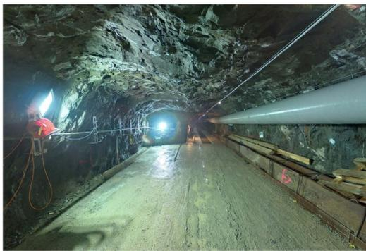
Figure 1: Impression from the new Bedretto Deep Underground Laboratory for Geoenergy Research. The lab provides unparalleled access to a large undisturbed rock volume in the widely homogeneous Rotondo Granite.
