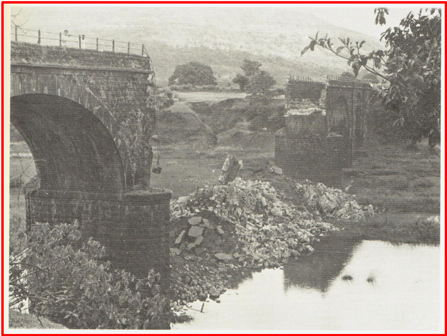
The stone masonry arch bridge on the Helwak-Chiplum road collapsed
