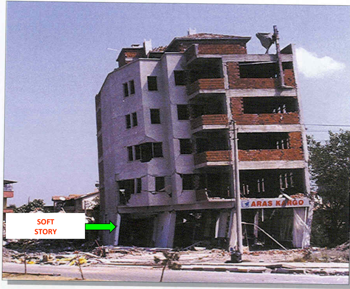
DAMAGE TO A TYPICAL APARTMENT BUILDING WITH SOFT FIRST STORY DURING THE M=7.4, 1999 KOCAELI, TURKEY EARTHQUAKE
