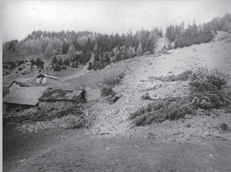
Many roads were cut off by the avalanches and landslides triggered by the earthquake. Today this kind of damage would have a major impact on the Valais economy for several months.
