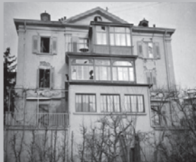
The inhabitants feared the buildings would collapse because of all the aftershocks. Would you still want to spend the night in this building?
