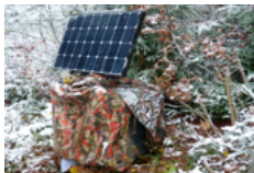
Solar-powered temporary seismic monitoring station in the geothermal energy project in St. Gallen
