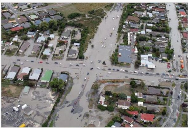
Water damage in on the corner of Pages Rd and ANZAC Dr.
