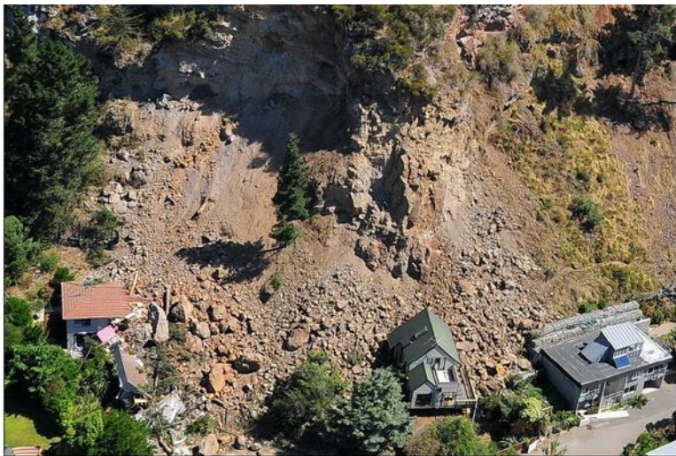
Photo 17. GTH_5787 - House destroyed by rock fall at 54 Raekura Place, Redcliffs (reported fatality site).
